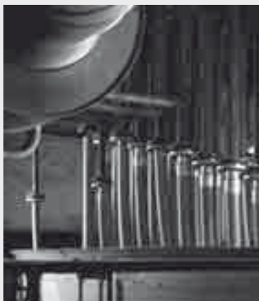
Metal hoses as flexible link between pipe and machine
